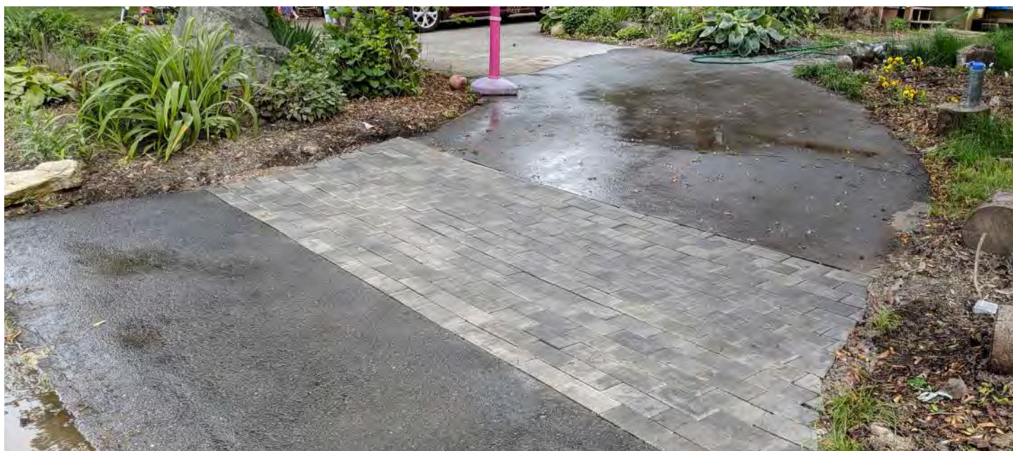
Pervious Driveway Installed on Aquidneck Island
