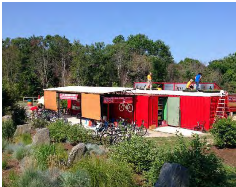
Installation of Green Roof on Red Shed Bike Shop
